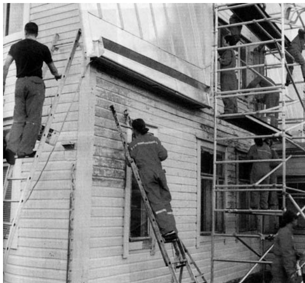
Oranssi tenants renovating during renovation
